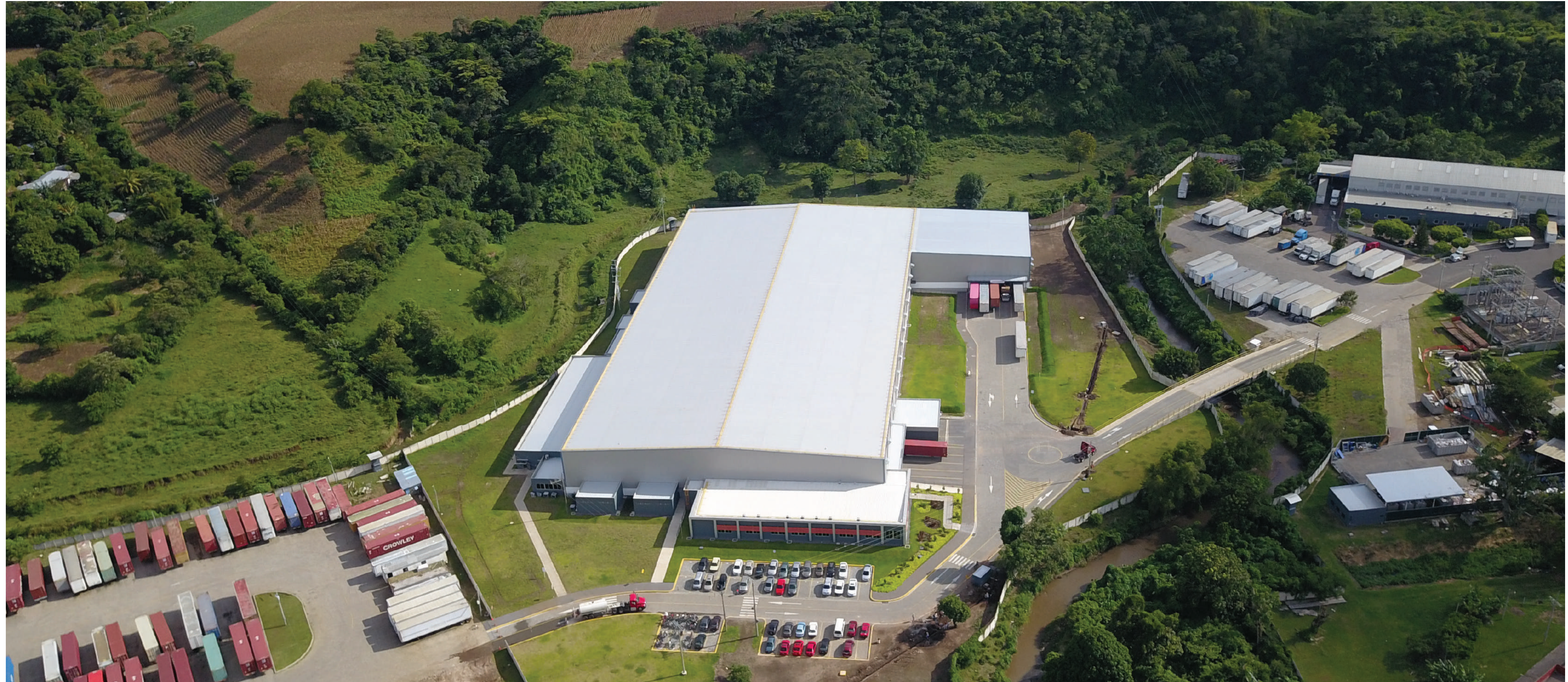
Block T / American Industrial Park
